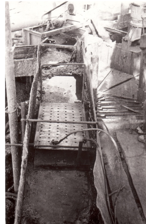
Since 1977 many drills on fields in South-Western Uzbekistan and Eastern Turkmenistan was equipped with devices UOBR for unipolar cathode processing of drilling mud. Due to these devices the consumption of chemical reagents – regulators of viscosity and water loss of a drilling fluid - was reduced by 30 - 70%. Uzbekistan, 1977.
